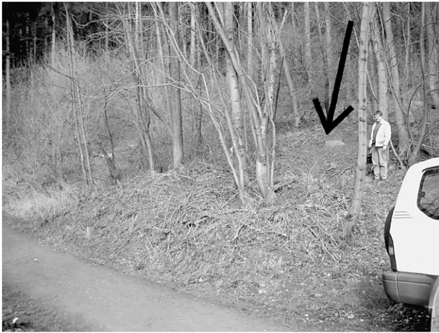
Fig. 2. Photograph of the section of the landslide that includes the monitoring station. The boxes on the ground between the trees, contain the platform and the borehole tiltmeter (black arrow). The track cuts through the landslide.
