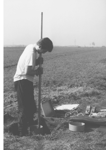
Figure A.4: Installation of a bore-hole tiltmeter by tampering, T4 OE .
