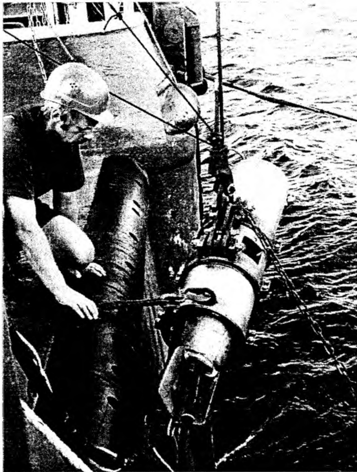
Figure 5.3.7: 32 l Bolt gun upon deployment onboard RV SONNE.
